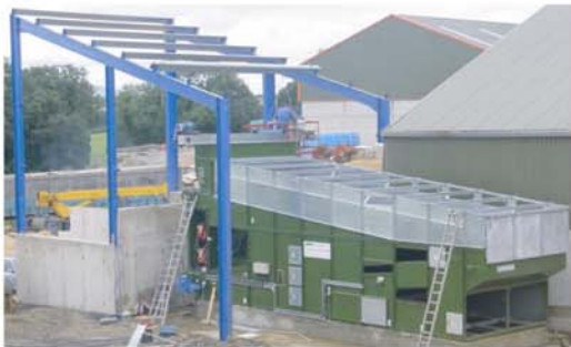
DF 30000 Drier - 33t/hr - during installation
